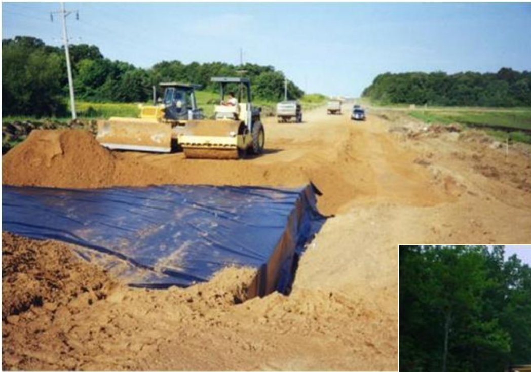
Adding Geosynthetic Liner and Covering Fill
